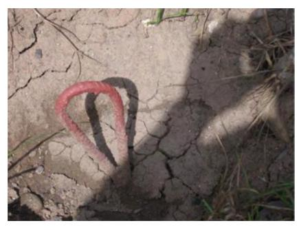
Fig. 3B Steel Cable used for Hurricane Straps
